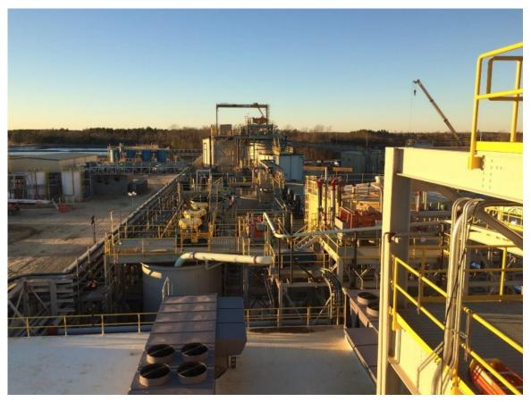
Figure A-48 Flotation and Ultrafine Grinding Circuit Source: Haile 2018.
