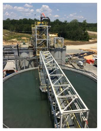
Figure A-56 Tails Thickener and Cyanide Destruct Circuit Source: Haile 2018.
