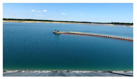
Figure A-68 TSF Reclaim Pond and Pumping Facility
