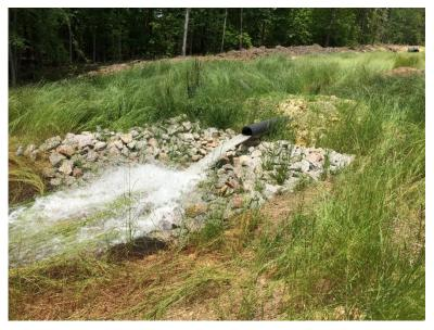
Figure A-74 NPDES 003 Outfall for Water Treatment Discharge Source: Haile 2018.
