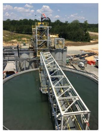
Figure A-54 Tails Thickener and Cyanide Destruct Circuit Source: Haile 2018.
