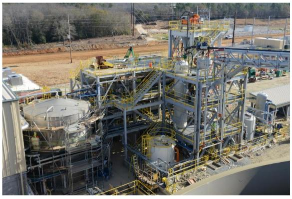
**Figure A-52** Elution Circuit – Acid Wash, Barren Tank, and Carbon Regeneration Rotary Kiln Source: Haile 2018.
