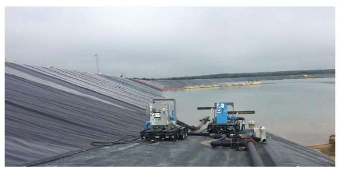
Figure A-66 TSF Reclaim Pond and Pumping Facility
