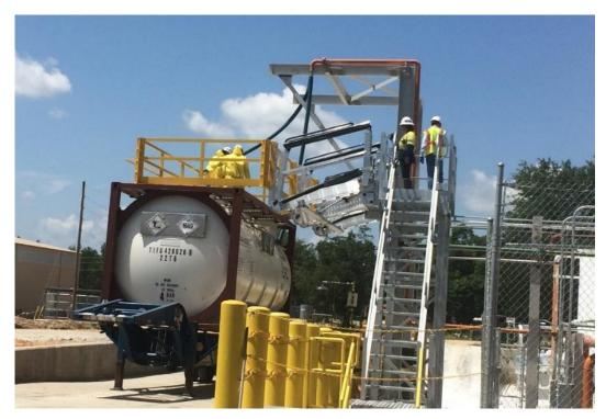
Figure A-53 Sodium Cyanide Transfer Station Source: Haile 2018.
