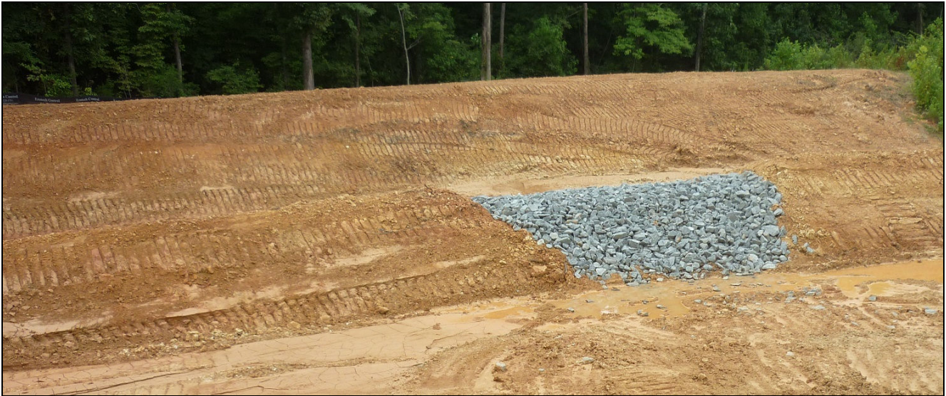
Photo: Sediment Forebay
