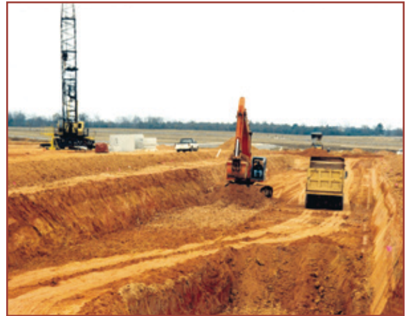
A typical B/C Trench under construction.
