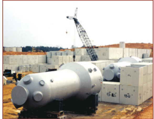
Low activity commercial reactor steam generators placed among disposal vaults for burial.
