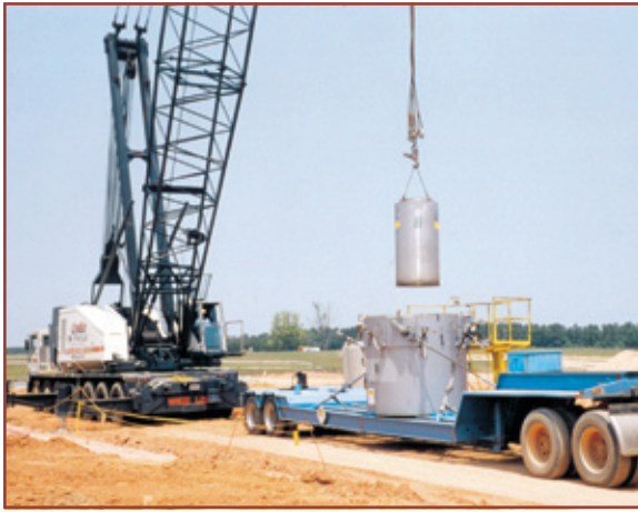
Transport Vehicle in position for removal of LLRW container prior to disposal in a B/C Trench.
