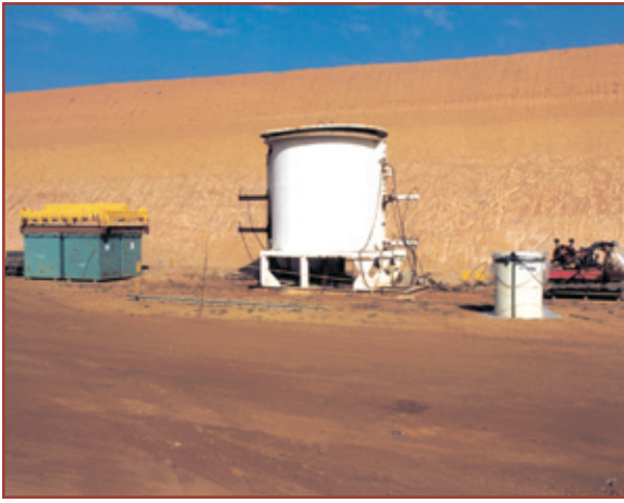
Hydraulic Liner and Drum puncture equipment is utilized to assure that no excessive liquids are present within waste packaging.
