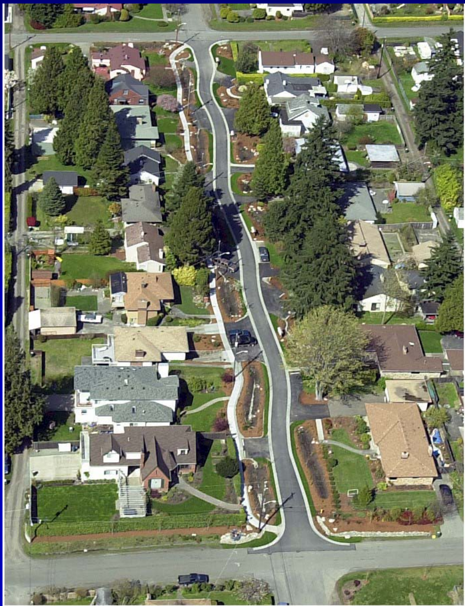
SEA Streets - After Construction 2nd Ave NW - NW 117th St to NW 120th St
