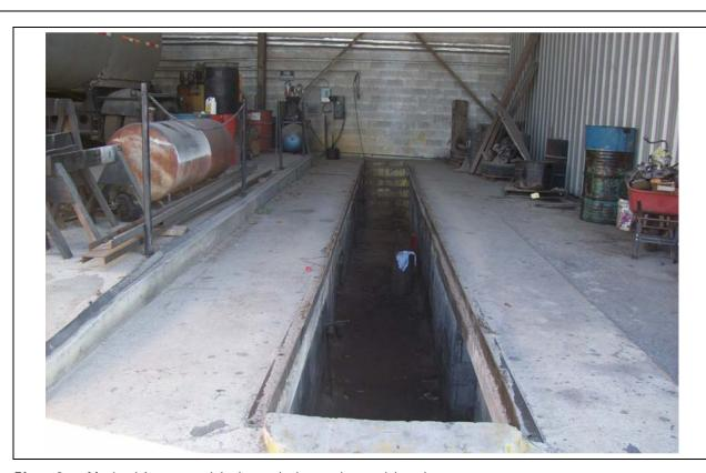
**Photo 8:** Mechanic's access pit in the truck shop at the emulsion plant.
