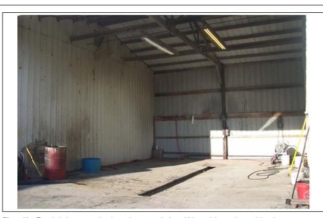
**Photo 10:** Trench drain connected to the sanitary sewer in the vehicle wash bay at the emulsion plant.
