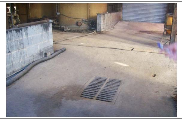
**Photo 11:** Storm water catch basin for the underground cistern located outside the northeastern portion of the mill building at the emulsion plant.
