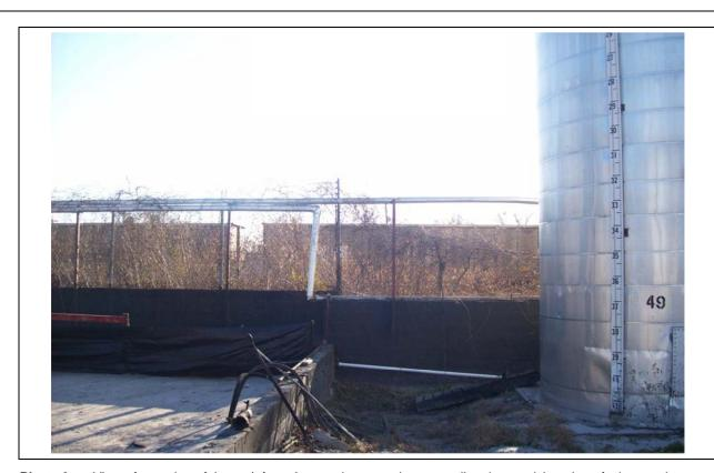
Photo 6: View of a portion of the tank farms' secondary containment wall at the emulsion plant, facing south.
